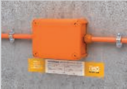
Fully installed FireBox with identification plate.
