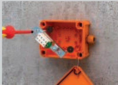
Mounting with fire protection bolt tie through the clamp and base of the FireBox.
